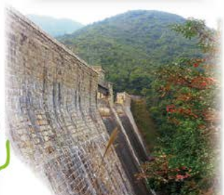
大潭中水塘水壩 Tai Tam Intermediate Reservoir Dam
