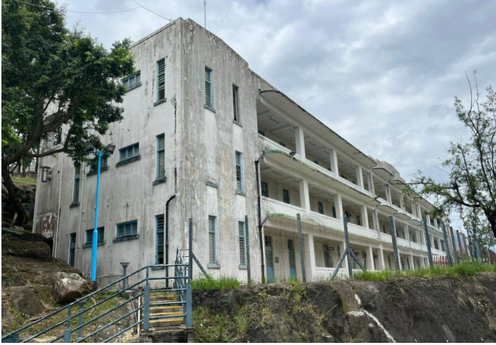
Block 5 — Assembly Hall
