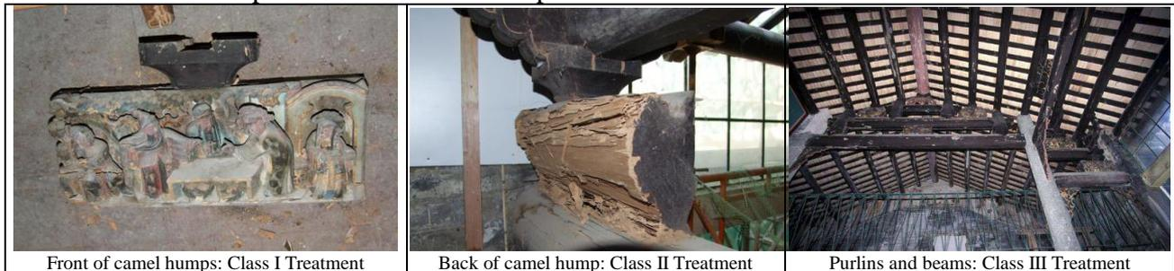
Fig. 2 Condition of wooden components before restoration
